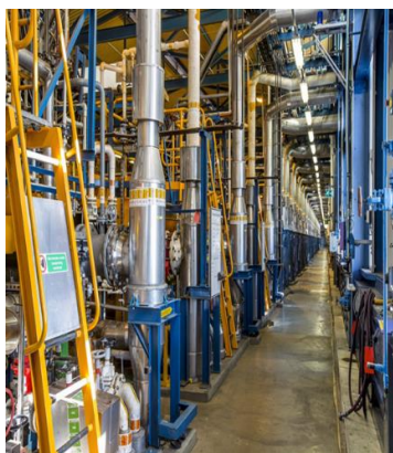
Figure 7.3: Electrolyzers for chlor-alkali production in Rotterdam
